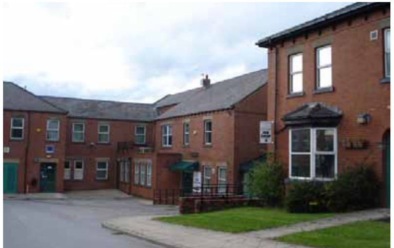
The Acorn Centre, housed in the old colliery offices Jenny Lunn © RGS-IBG Discovering Britain
