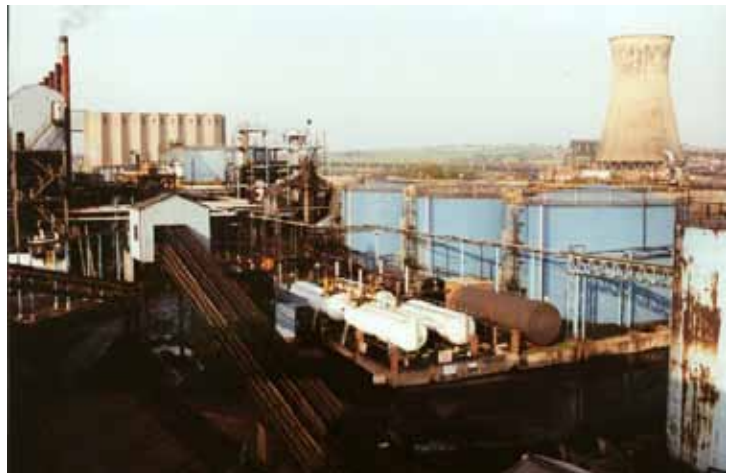
An industrial landscape From the Brierley Grimethorpe and Shafton Living Archive
