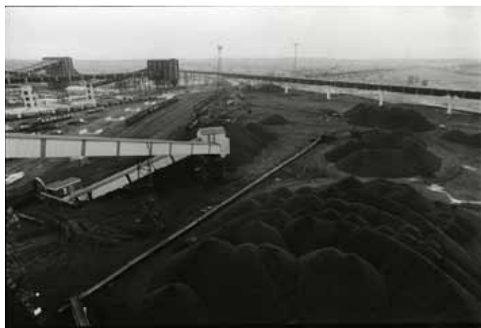
Coalite Coke Plant (1983) © Ross Williams Courtesy of National Coal Mining Museum of England
