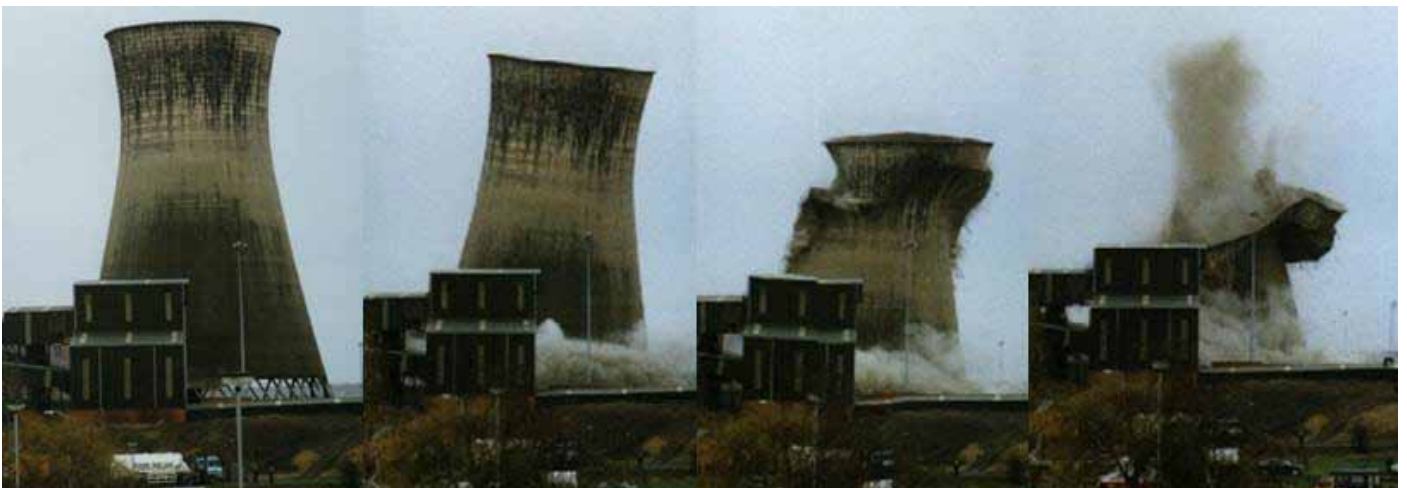
Clockwise from top left - clearance of the colliery site, sale of colliery buildings and demolition of the power station cooling tower From the Brierley Grimethorpe and Shafton Living Archive
